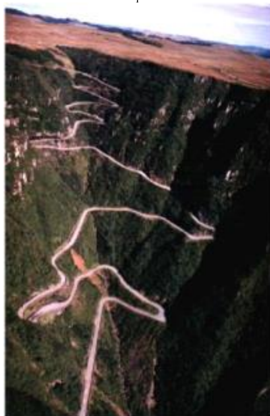
Figure 19 - SC-438 road from Lauro Muller to- São Joaquim and the top of the Serra do Rio do Rasto.
